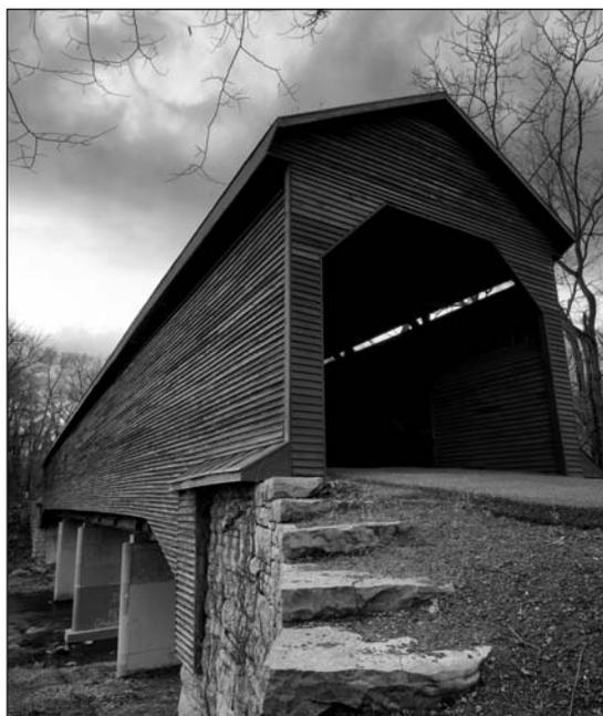
*Meems Bottom Covered Bridge in Mt. Jackson, Va. Built 1892-93 with a span of 200 feet, the bridge is supported by a Burr Arch and crosses the North Fork of the Shenandoah River. Meems Bottom is the longest remaining covered bridge in Virginia and the only covered bridge in the state that is open to vehicles. Photo by John Walrath.*
