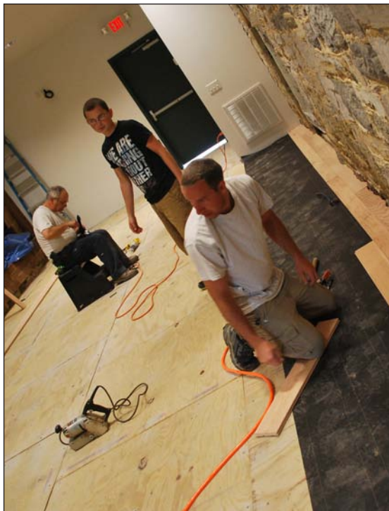
Lowe’s Heroes workers, left to right, Jeremy Mays, Jeff Poffenberger & Paul Mays helped to expertly install wormy red oak floorboards in the converted wagon shed room. Photo by Tracy Holliday.
